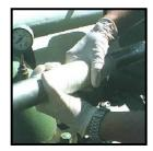
By utilising UPS Pipe Repair Tape – immediate and cost effective repairs can be carried out.
