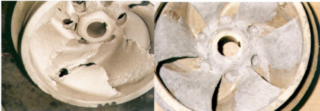
Pump Impeller blasted and then degreased with Unique Polymers Universal Cleaner. The damaged blades rebuilt with UPS 200 Ceramic Carbide Wearing Compound
