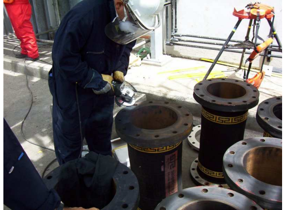
Surface Preparation Grinding
